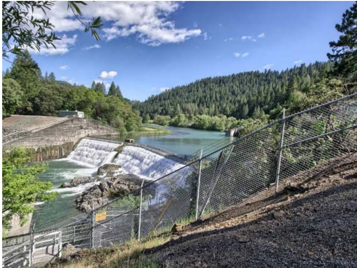
VAN ARSDALE FISHERIES STATION/RESERVOIR
